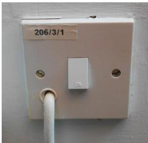
There is an ON/OFF switch located on the wall. Always leave the wall switch on as the heater may take 24 hours or overnight to operate.
